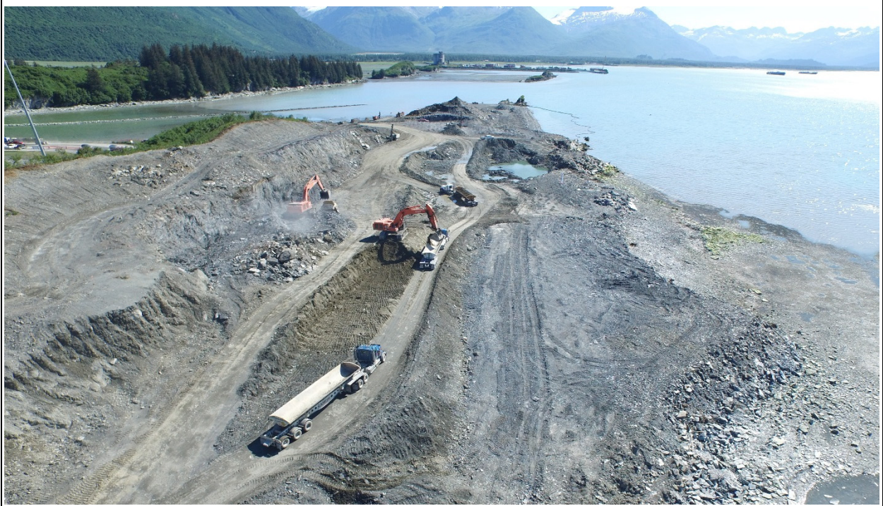
View West. Hill excavation in process along middle of the site; shot rock being loaded into wiggly wagon (left center) for stockpile at Sea Otter; overburden (center) being loaded into side dump trucks for City sites. (Talbot)
