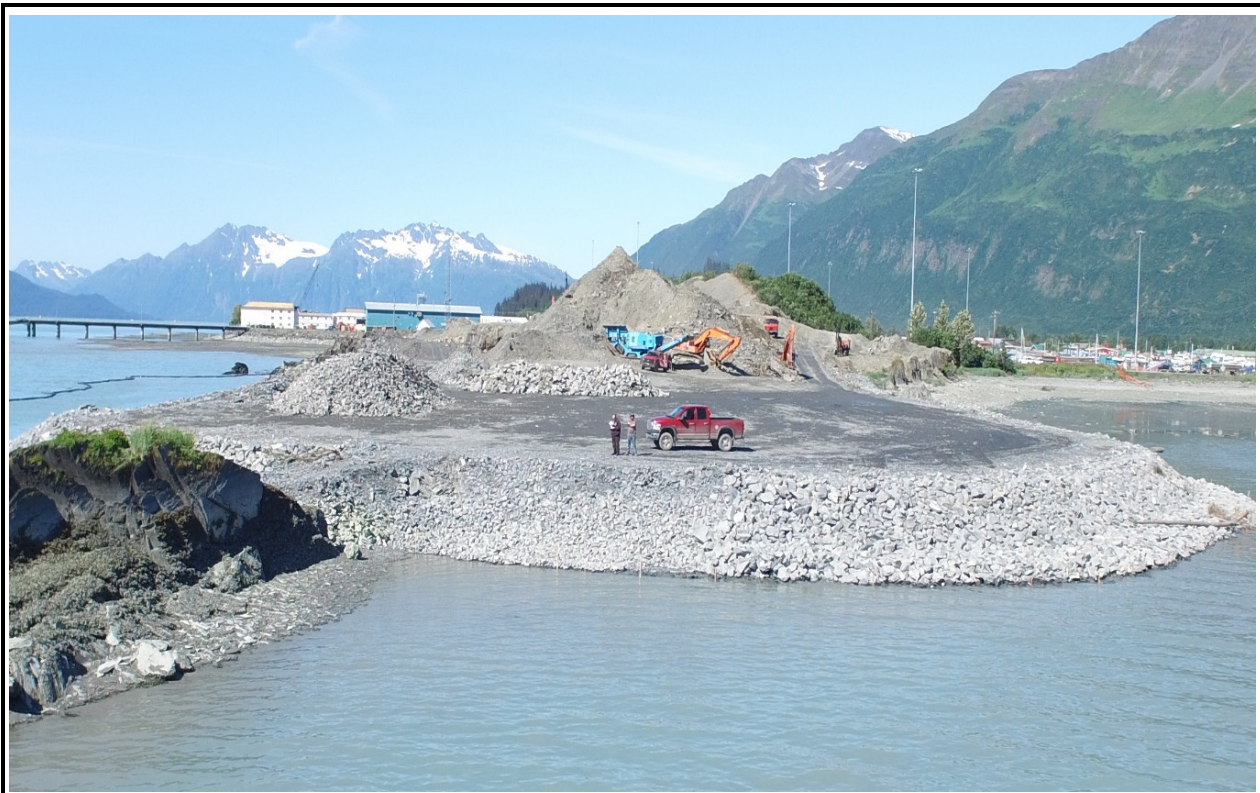
View West. East fill has been constructed to 10 foot elevation except along south side, with filter rock and riprap placed on most of the north and east slopes. Stockpiles on the fill contain filter rock and riprap (by J. Talbot, COV)
