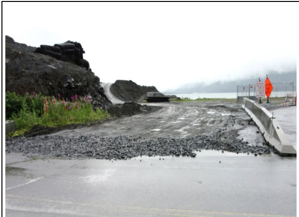
Rock (left) was shot, excavated and graded for West access
