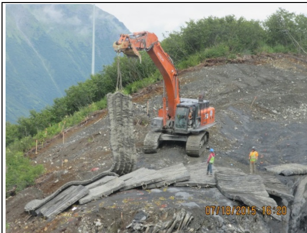
Heavy mats are placed over blast area to prevent "fly" rock
