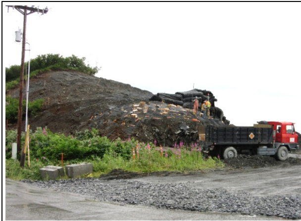
Advanced Blasting crew staging and loading explosives
