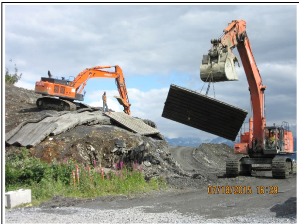
Timber panels also placed to prevent "fly" rock
