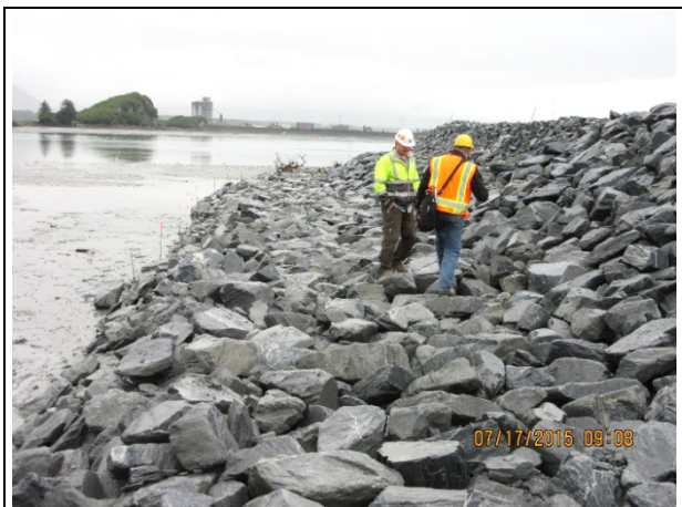
Engineer inspecting riprap placed at north toe of fill slope
