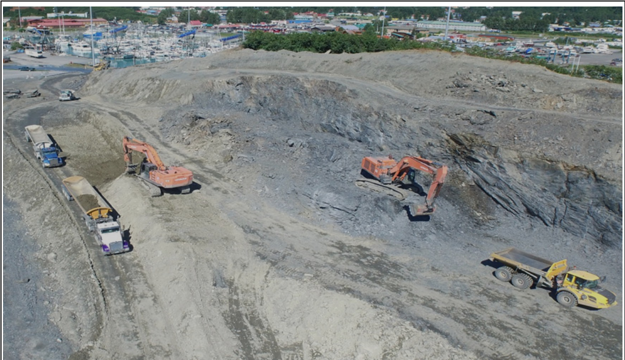
View NW. Rock excavation (right) and overburden (left) at same location as above photo. Blasting and excavation created construction access at west end to South Harbor Drive (upper left) next to SERV'S parking lot. (Talbot)
