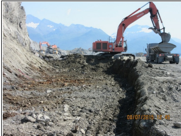
Ground view of 4' sub excavation to remove silty soils
