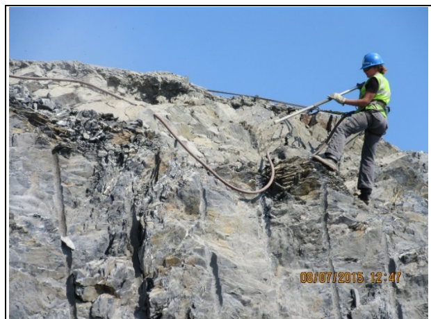
Removing loose rock (scale) at top of slope with air knife
