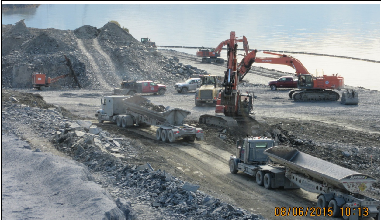
View East. Last of mass excavation in process near east end of Hotel Hill. Loading side dumps with overburden (front) for hauling to City C&D Pit. Crusher beyond mound at upper left. South edge of east fill at upper right.
