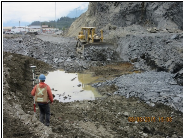
Shot rock backfill in bottom of 8' subex for wash-down pad
