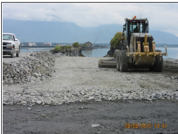
Grading 12" lift of crushed material on fill at 10' elevation
