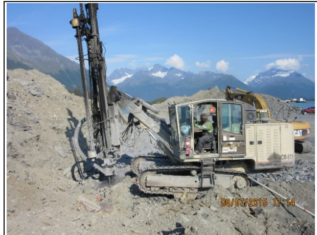
Drilling rock near east end for blasting to subgrade
