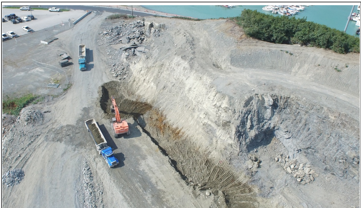
View Northwest. Excavating frost-susceptible soil 4' below subgrade near future west entrance. The wash down pad, also in this area, was excavated 8' below subgrade. Scaling top of the slope at lower right (J. Talbott, COV)
