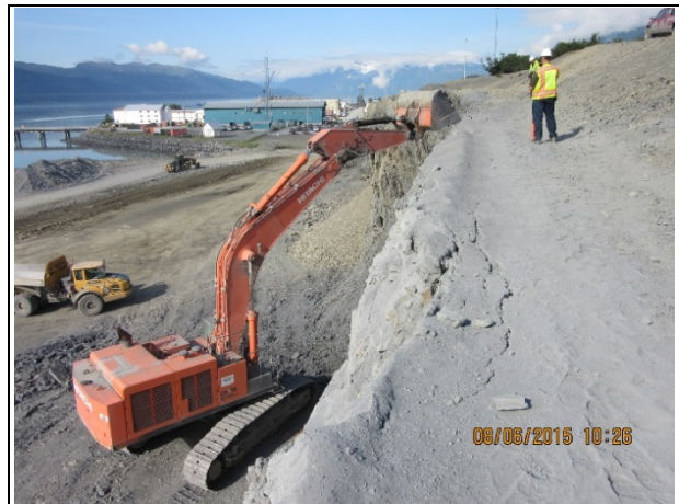
Excavator carefully removing loose rock at top of slope
