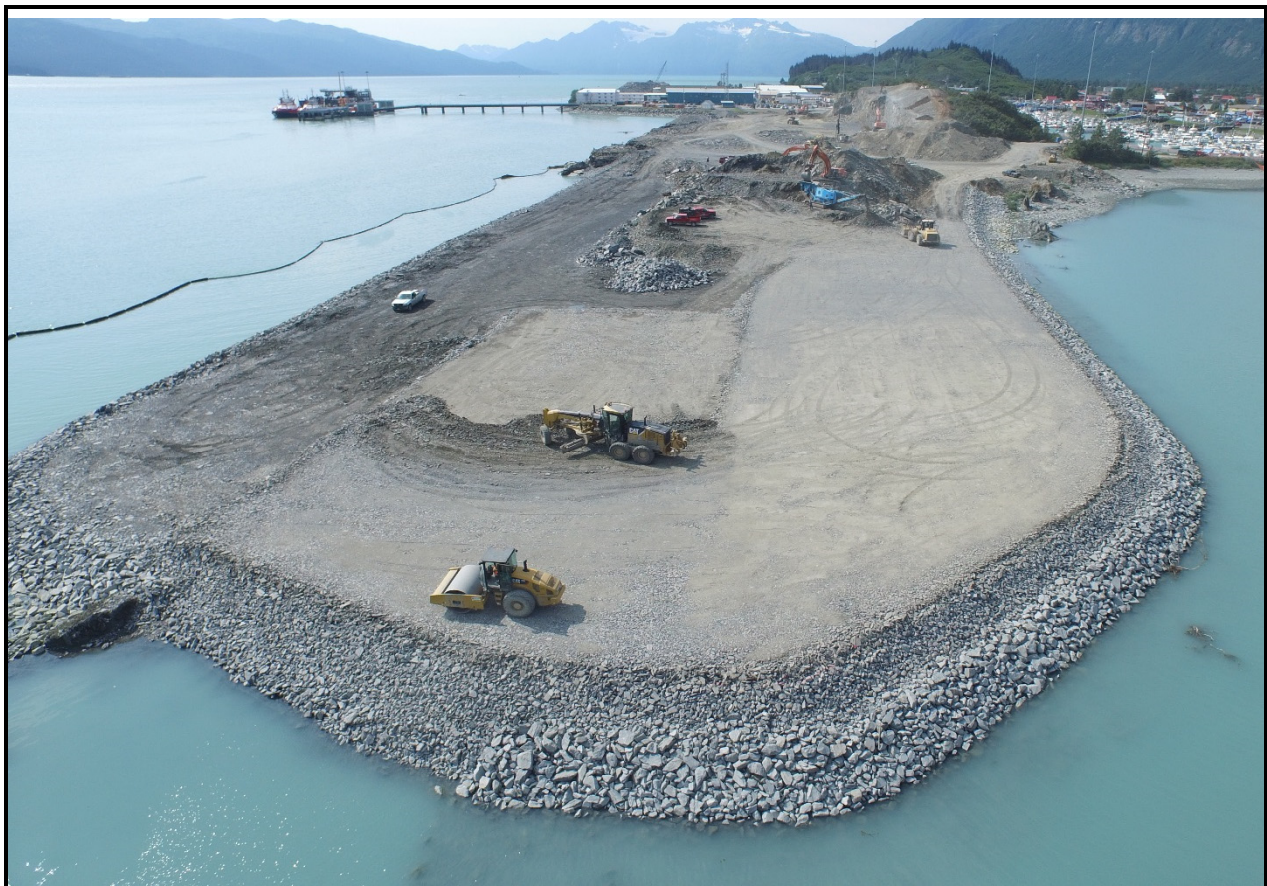
View West. East fill is being constructed with 12" lifts of processed material above 10' elevation, with filter rock and riprap placed on the slope. Grader spreads and vibrator roller compacts each lift. (by J. Talbott, COV)
